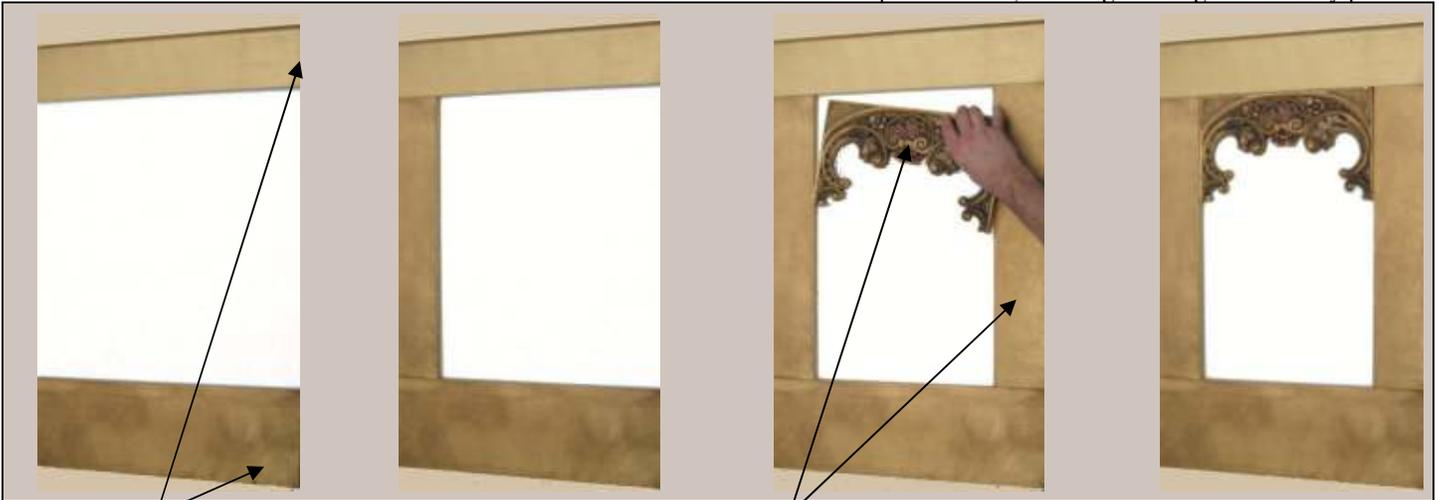
Install 8"x3/4" MDF base-board, and 5"x3/4" MDF chair rail base over drywall along the entire wall.
