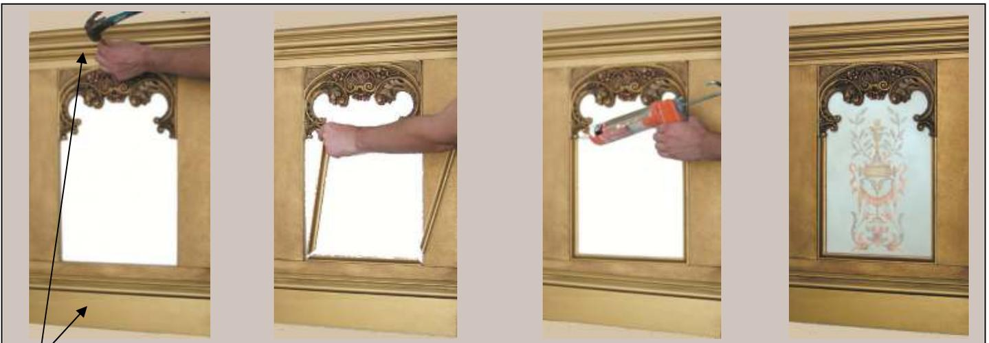
After panel tops & spacer boards are up, nail chair rail & base molding over MDF bases. Use adhesive caulk and a few finishing nails to attach each of the two moldings in place.
